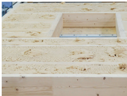
Wide range of insulation materials , such as cellulose, wood fiber, mineral wool can be insulated.
